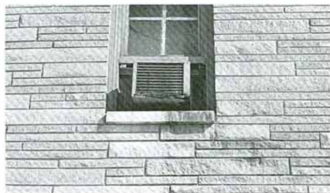
Lack of maintenance on this air conditioner has produced a badly stained sill and other stones in the splitface wall below.
