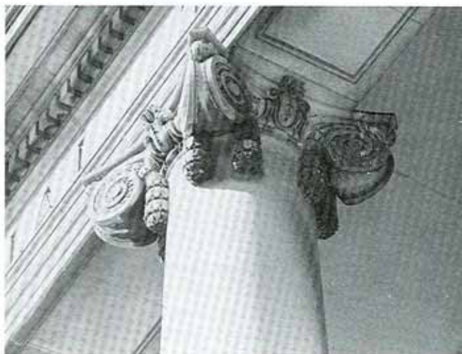
The lower areas of the volutes on this Ionic cap are protected from weathering. The resultant encrustation from years of soot could be greatly lightened if not entirely removed by scrubbing.
