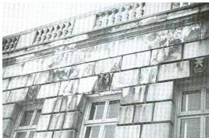
A badly leaking roof caused this eyesore. When the leaks were repaired, the efflorescence cleared up within a few months.
